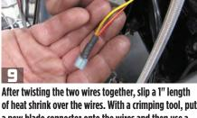
of heat shrink over the wires. With a crimping tool, put a new blade connector onto the wires and then use a heat gun to shrink the tubing.
